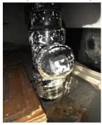
Basement Floor Drain: corroded strainer - replace
