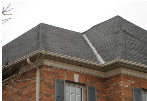
loose shingle at rear garage
