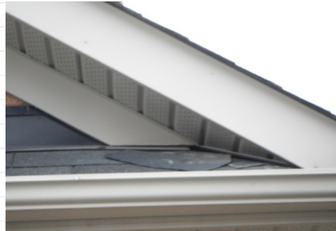
loose shingle at rear garage
