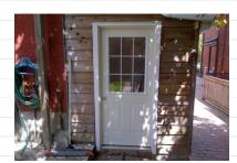
Door: 2nd level rear - missing rail - unsafe condition
