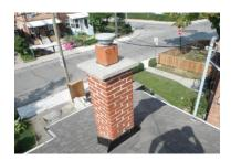
South: masonry has been 'patched' with parging, monitor and repair as required
