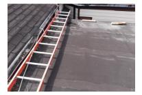
2nd Slope: lower north: low slope roof therefore replace with modified bitumen requires maintenance against wall
