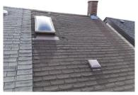
Flat Surface: low quality materials/installation, presently requires maintenance, recommend replacing with modified bitumen (rubber)
